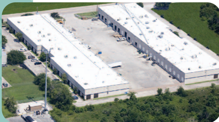
ABM INTERNATIONAL'S WORLDWIDE HEADQUARTERS, HOUSTON TEXAS
